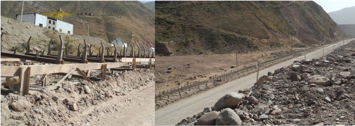
Figure 6-1 : Remains of the conveyor stretches already installed
