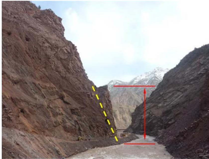
Figure 3-5 : Central core area excavations
