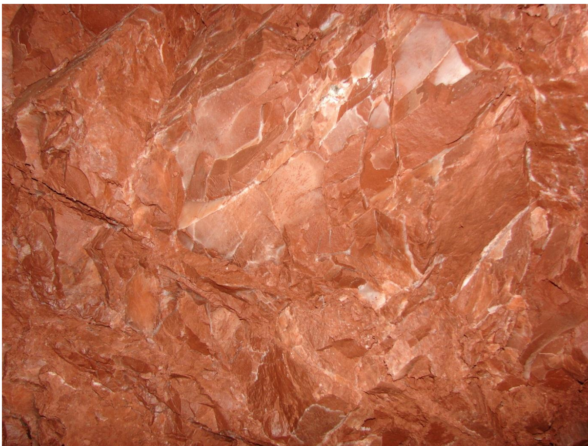
Figure 8.3: Close view of Gaurdak claystone and quasi-systematic, fine gypsum encrusting of discontinuities (gallery 1034)
