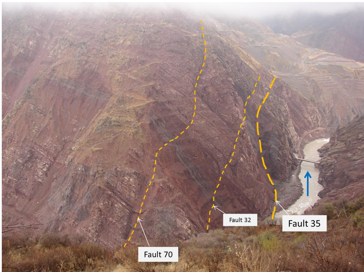
Figure 2.3: View of the gorge of Vakhsh River on the dam site, towards downstream; Fault 35 is highlighted in the left bank, as well as approximate traces of Fault 70 and the minor Fault 32 (named as per original drawing 1174-03-78, Sheet 1 of Ref.[1]), both of them of similar attitude; the dam axis is near to the intersection of Fault 35 and the river bed
