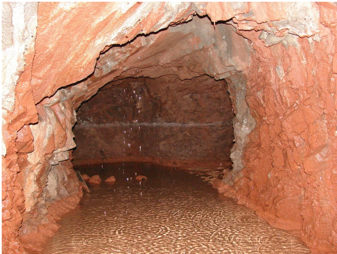
Figure 8.5: View of water circulations within a branch of investigation gallery 1002; red clay is clearly seen being taken along by water along the joints, then depositing on the floor
