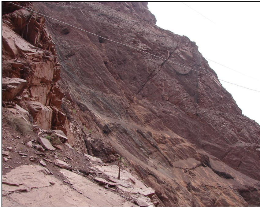
Figure 8.8: Fault of similar attitude as Fault 35, dipping towards upstream, cutting the Lower Obigarm siltstone and Upper Obigarm sandstone; in the background; other joints pertaining to the same system are clearly visible (bedding attitude steeply dipping towards upstream)
