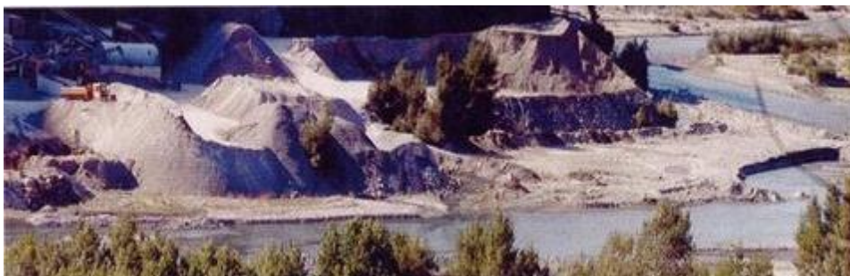
Figure 6.5 : Coarse sediment removal of the Sautet dam (France)
