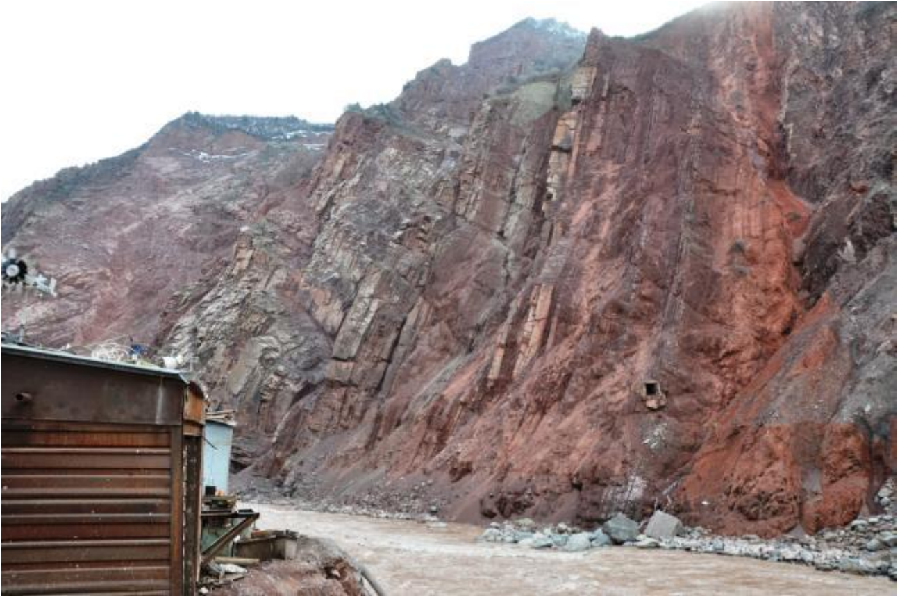
Illustration no. 23. Series of discontinuities of F#35 family I the Right Abutment.
