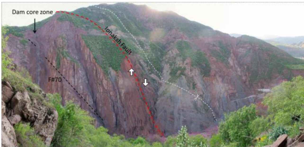
Illustration no. 15. Right Bank at the dam site
