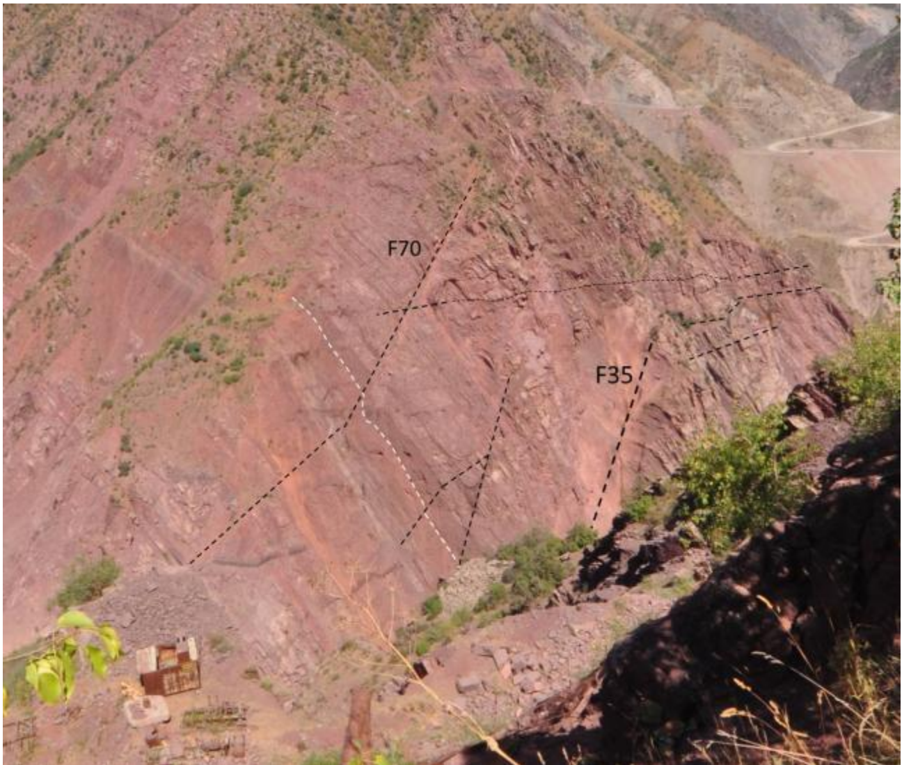
Illustration no. 25. Faults in the upper Left Abutment.
