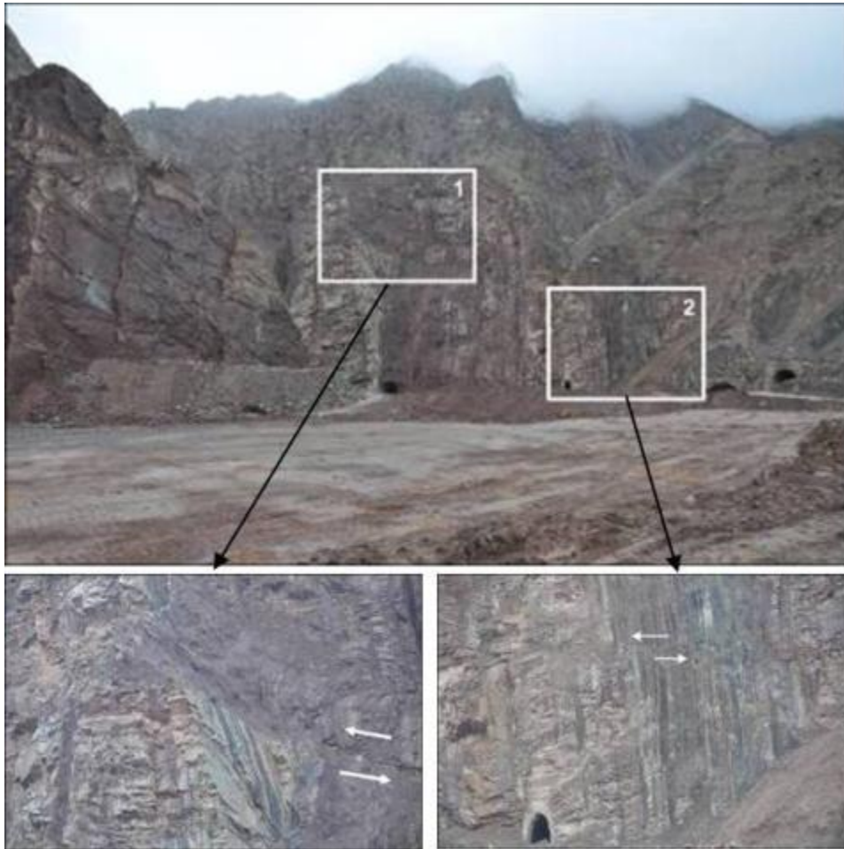
Illustration no. 28. Offsets on very persistent subhorizontal / shallow dipping discontinuities, Left Bank downstream.
