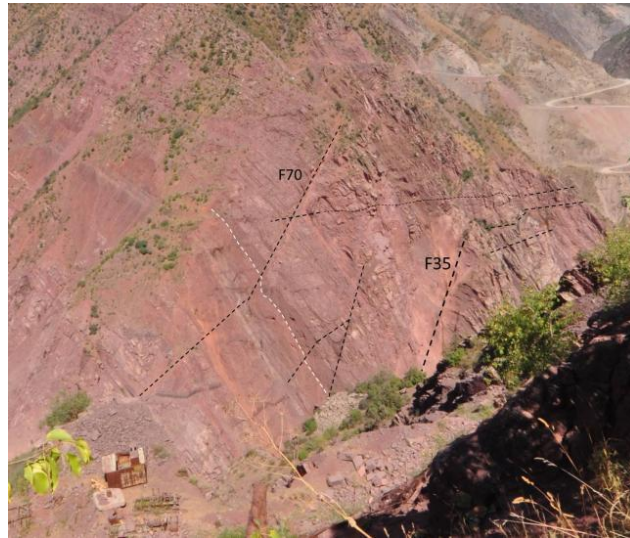
Figure 11 - Faults #35 and #70 in the upper Left Abutment. Location on Figure 10.
