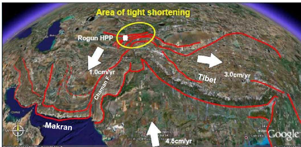
Figure 2 - India-Asia collision and induced deformation within Eurasia. Note that the Rogun HPP is located within the western syntax of the Himalaya, which is characterized by intensive shortening. White square shows the Rogun dam site.
